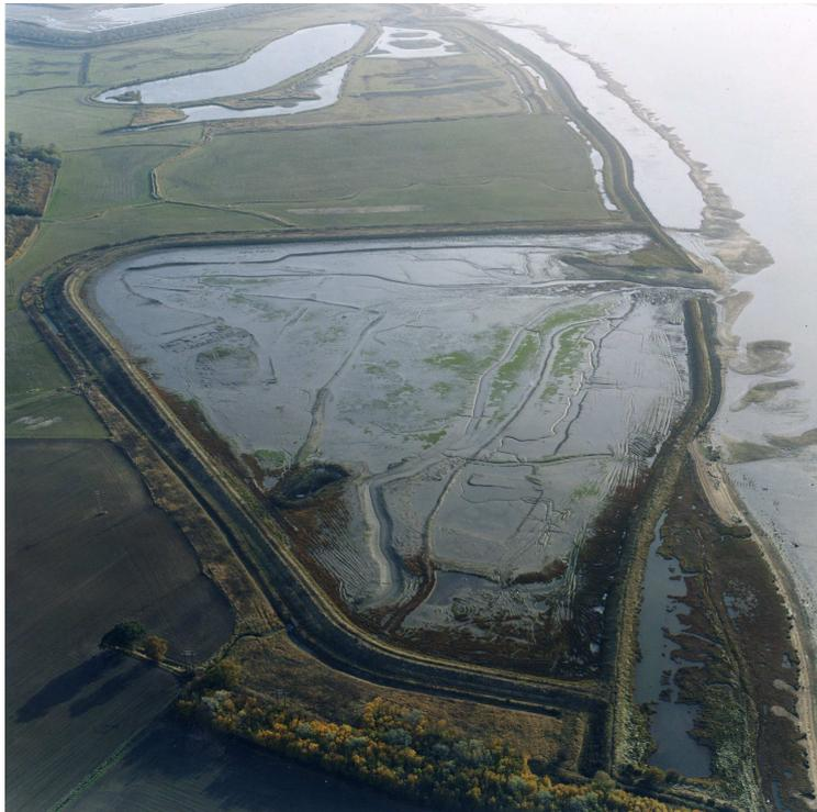
**Photograph 6.2 Aerial view of the 16.5ha Trimley managed realignment scheme on the eastern shore of the Orwell estuary, looking north-west (source: HHA)**
